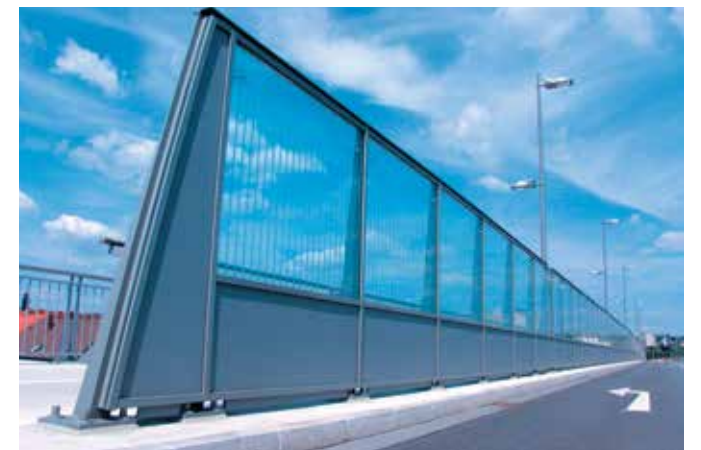
Noise barrier, Nibelungenbrücke, Regensburg Lower part made of PLEXIGLAS® Soundstop NT Fa. Markus Kaiser
