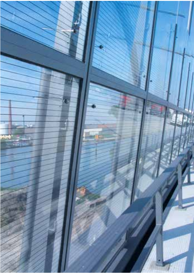
The uppermost PLEXIGLAS® SoundstopGS CC elements are partially freestanding.
