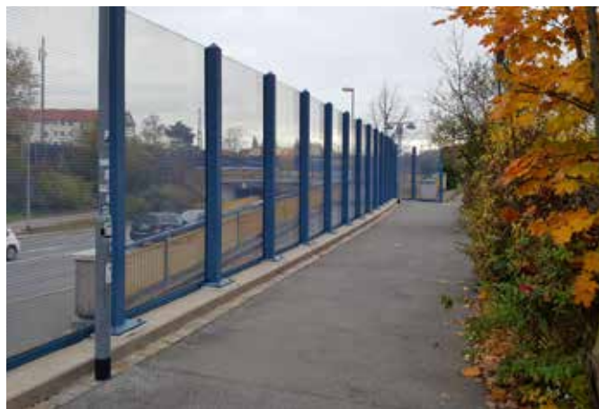
Noise barrier, Pollenfeld PLEXIGLAS® Soundstop XT BirdGuard, 20 mm
