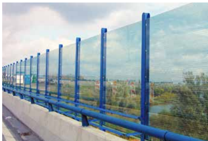
Noise barrier, Praha 6, Ruzyne PLEXIGLAS® Soundstop XT SMP Construction a.s.
