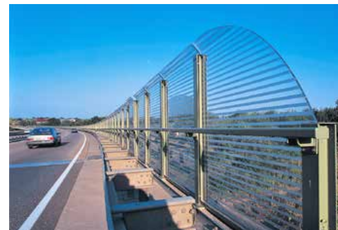
Noise barrier, Eltville PLEXIGLAS® Soundstop XT
