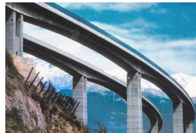
Noise barrier, Bridge Turin–Frejus PLEXIGLAS® Soundstop XT Tubosider ITALIANA S.p.A.
