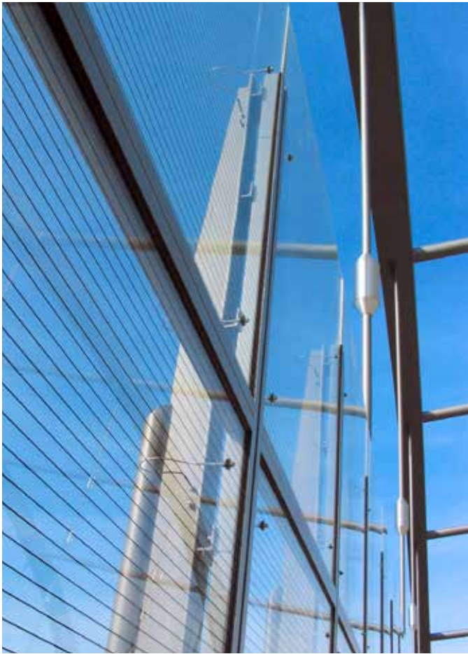
Detailed View The inclination of the noise barrier follows the inclination of the bridge structure (inclined inwards by 10°).
