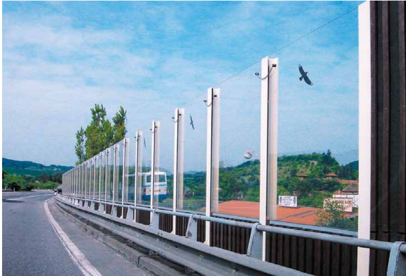
Noise barrier, Motoway D5, Lodenice PLEXIGLAS® Soundstop XT Stavebni technologie
